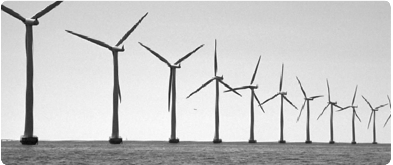
Middelgrunden wind farm, Denmark
