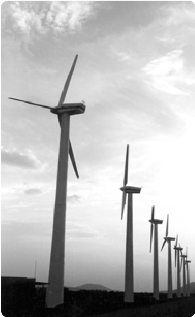
E. La Venta wind farm, Mexico
