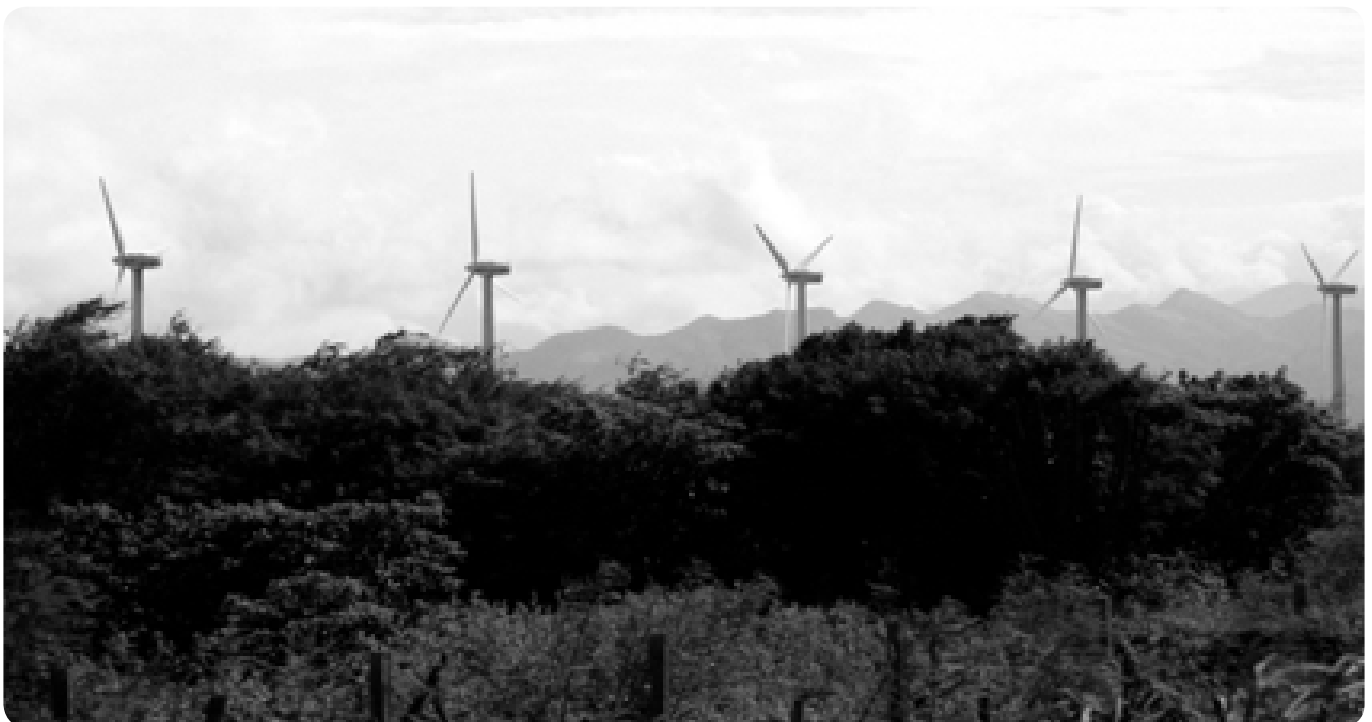
E. La Venta wind farm, Mexico
