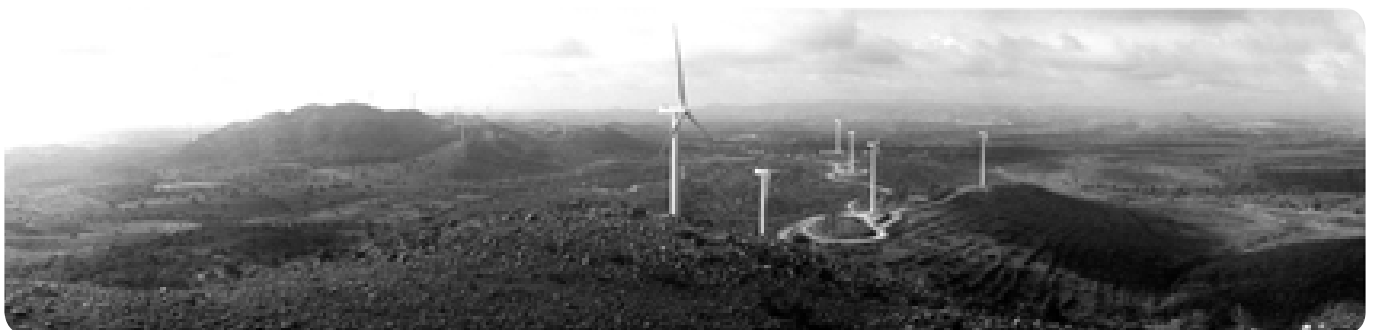
GR Halli wind farm, Karnataka, India
