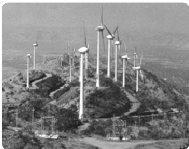
Chitradurga wind farm, Karnataka, India
