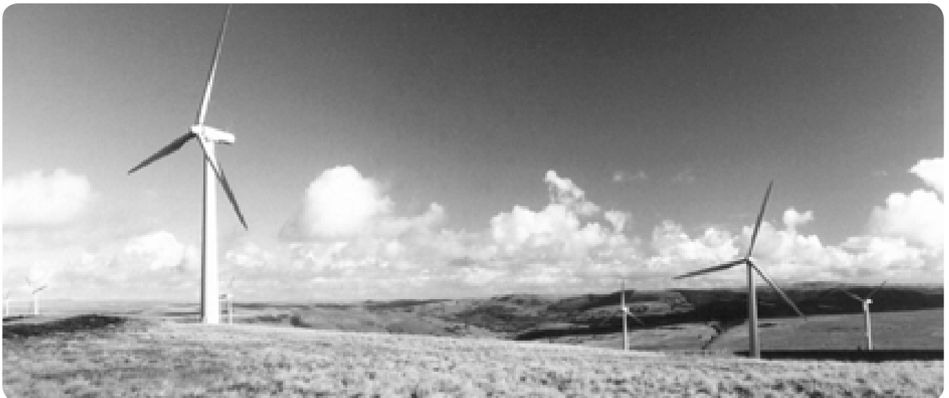
Carno wind farm, Wales, UK
