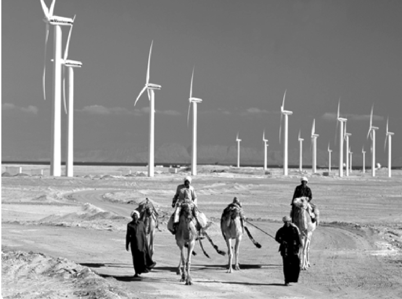
Zafarana wind farm, Egypt
