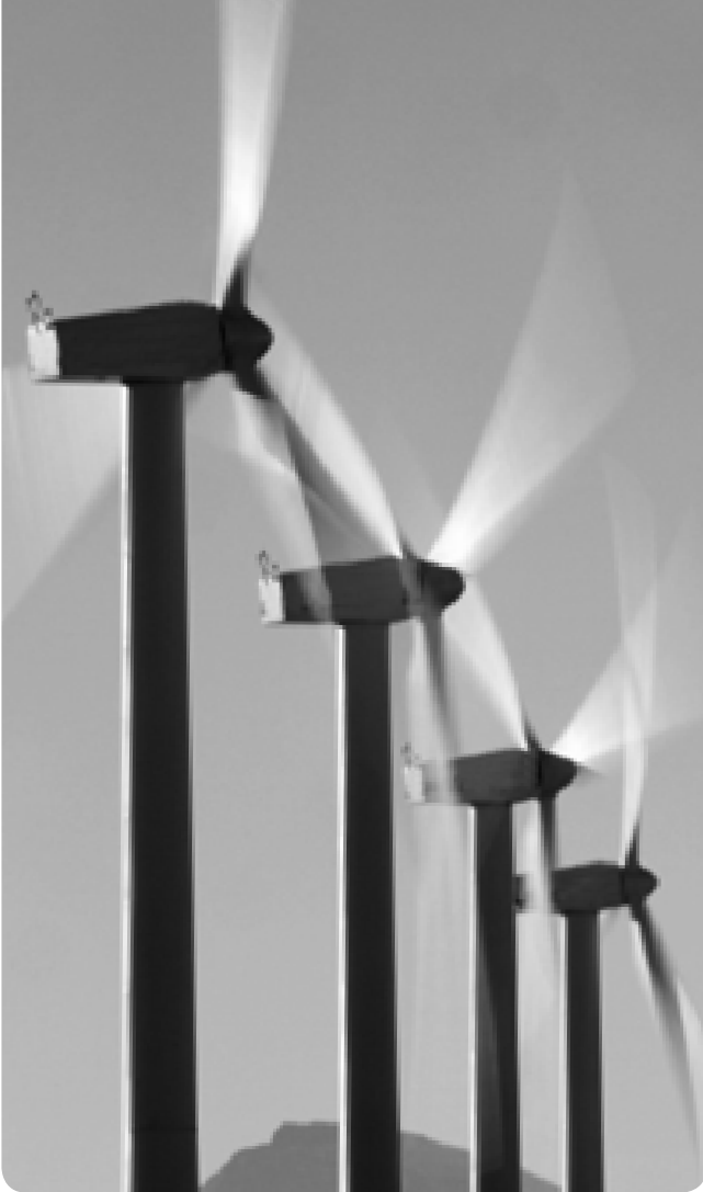
Castle River wind farm, Alberta, Canada
